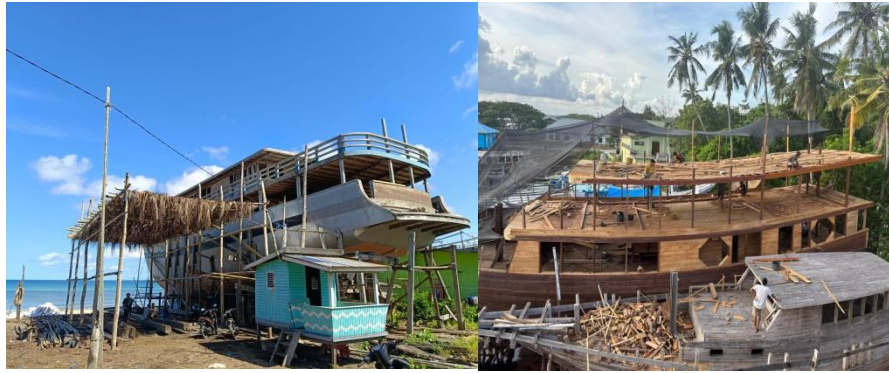
Figure 2. The Process of Making a Pinisi Ship Hull
