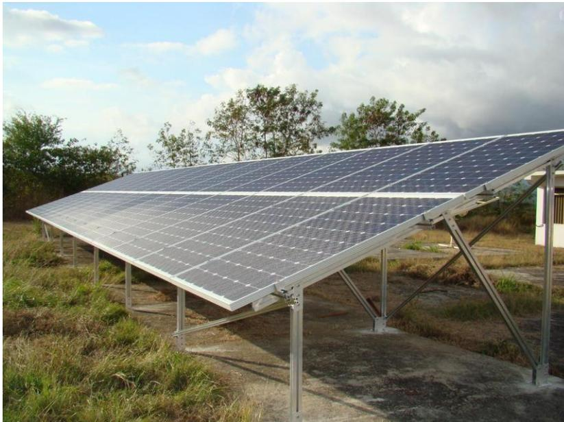
*Figure 1. PV Microsystem 7.5 kWp*
